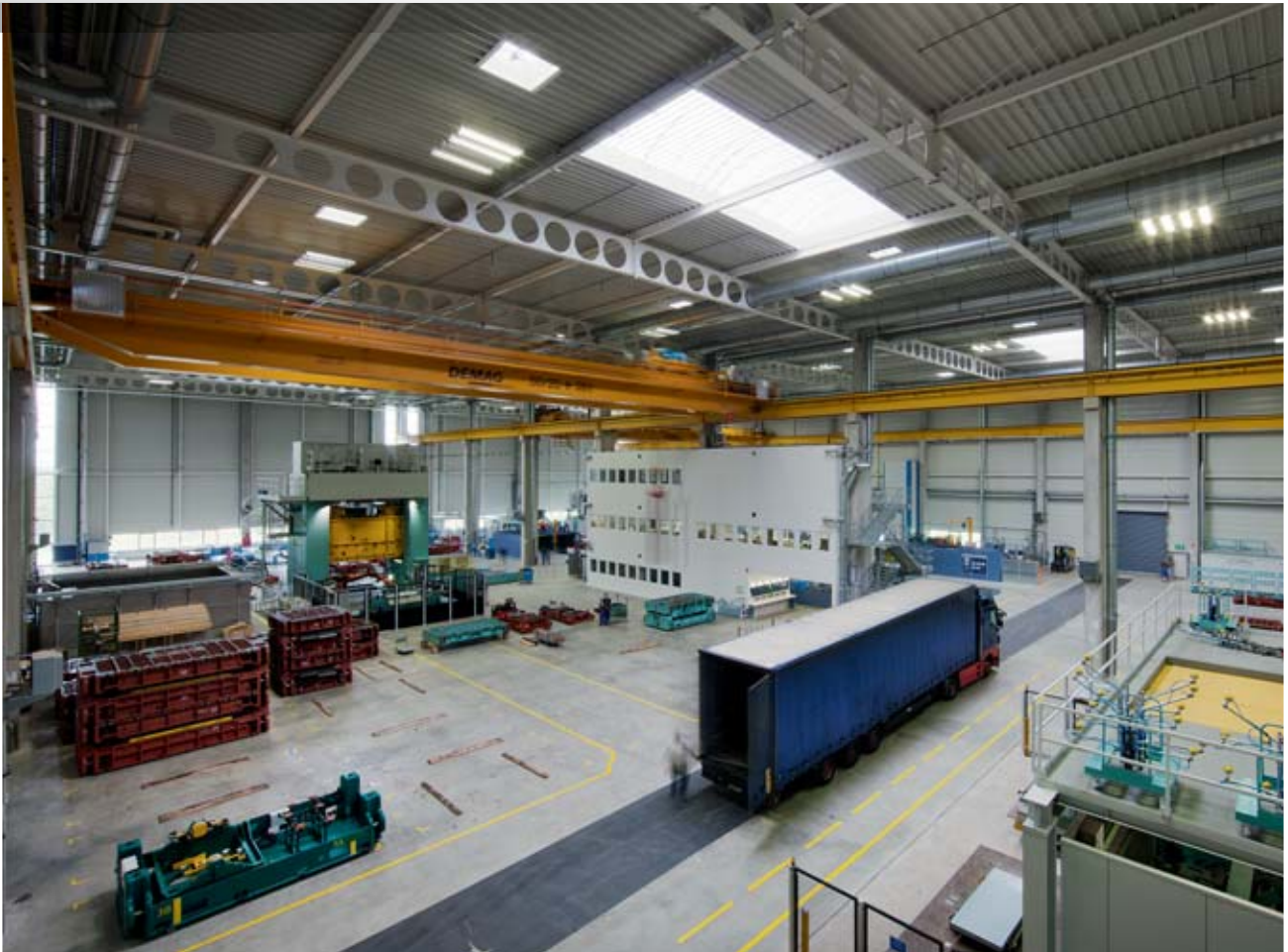
Oversize machines for manufacturing the car parts are arranged on both sides of the way through the press and coil hall.
