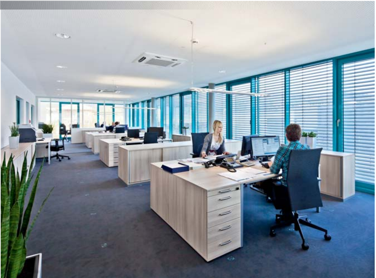
Neximo suspended luminaires as well as Athenik and Inperly downlights by TRILUX ensure well-balanced general and targeted lighting of the workstations in the open-plan office area of the administration wing.
