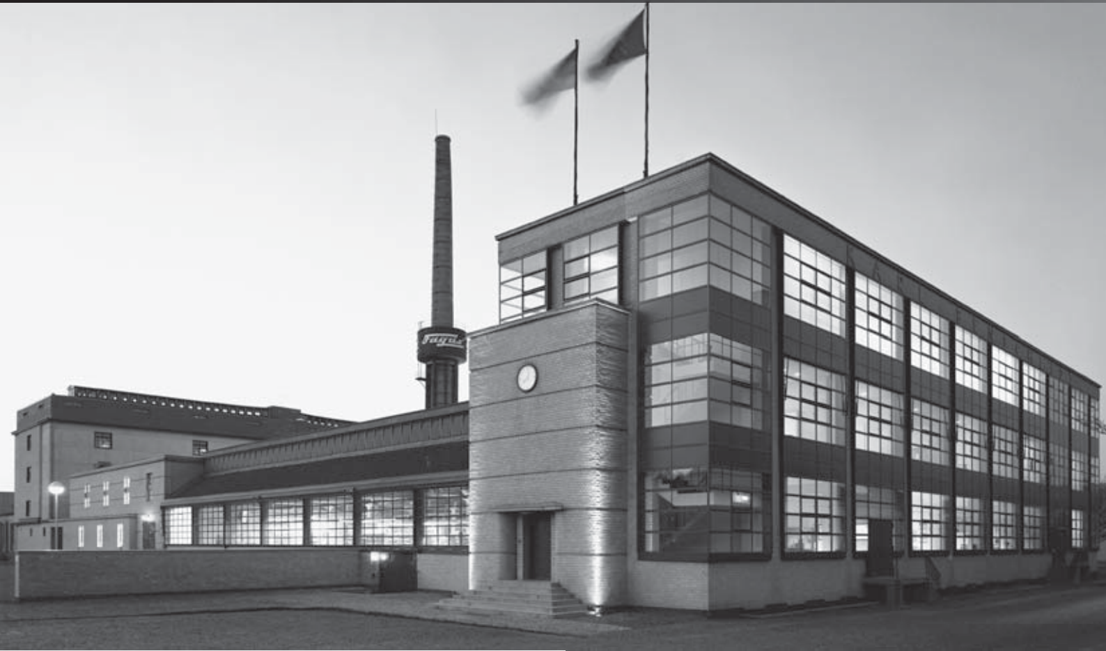
Fagus works, Karl Benscheidt footwear lasts manufacturing plant in Alfeld-an-der-Leine, built in 1911 to designs by Walter Gropius and Adolf Meyer, to this day a production location.
