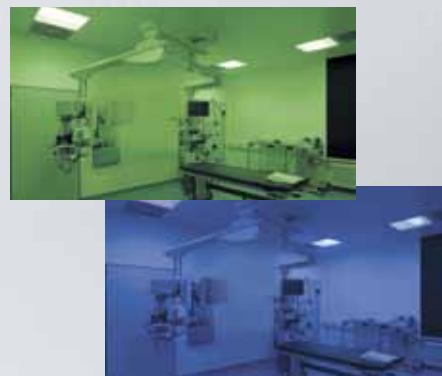
Colour scenes and colour temperatures can be individually set, sequences according to time of day are possible and supplementary areas can be controlled individually.
