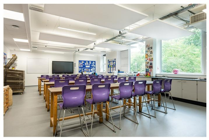
In the teaching spaces, each luminaire row is independently controlled via manual inputs and the automatic system. Additionally, emergency lighting versions of the standard luminaires were chosen to provide the required minimum lighting levels in a power failure.
