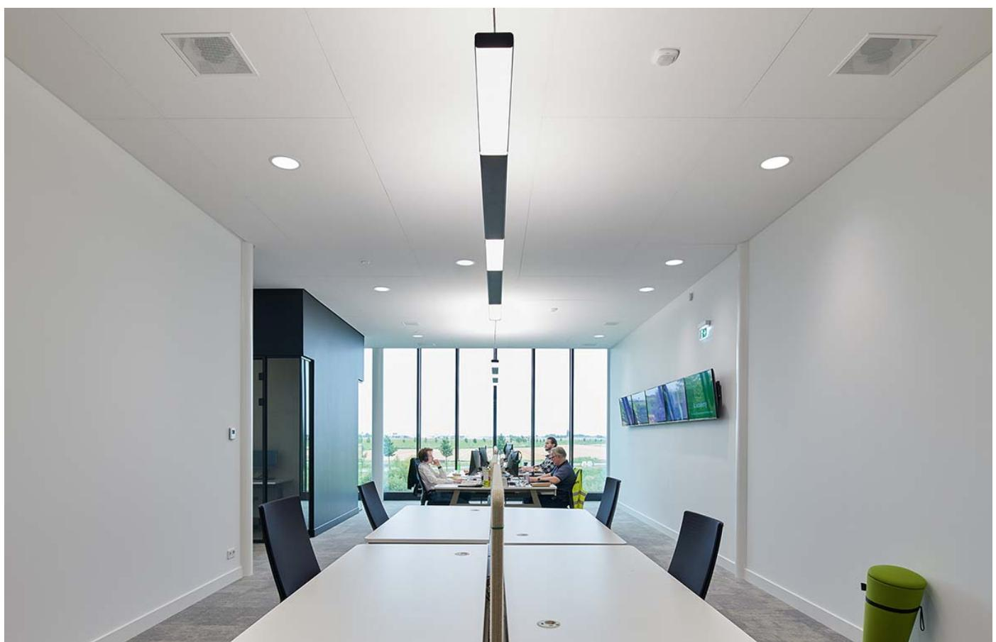
Indirect lighting at the workspaces is provided by pendant LED luminaires, creating a pleasant and spacious atmosphere. Elegant, long light strips provide general lighting, combined with LED spots for accent lighting. Cove lighting in the daylight domes enhances the effect of the staircase and the dome, completing the overall lighting design.
