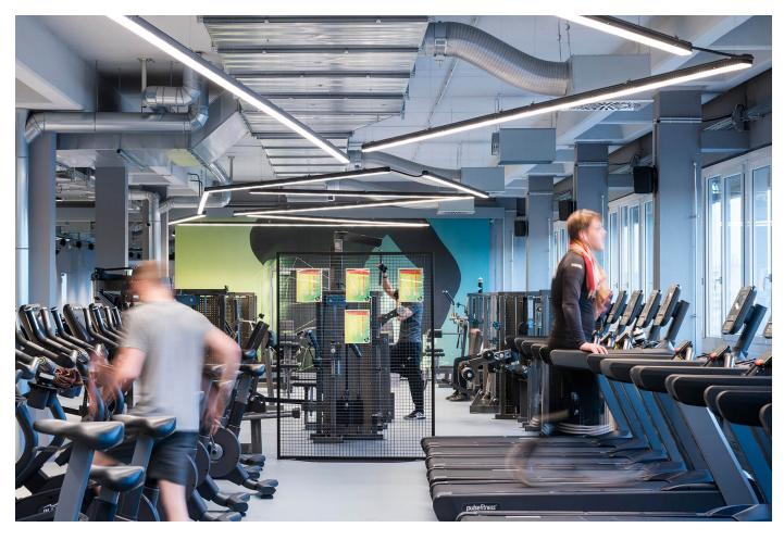
The areas of cardio and equipment training were equipped with the flexible light strip system E-LINE. In the room the light strips are arranged in the shape of a polygon – in that way, they support the company's CI and enliven the area.
